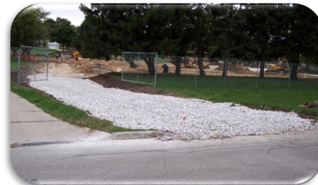
Stabilized stone construction entrance. For more information about use and installation see the "Construction Site Entrance" brochure or contact the Stormwater Department.
